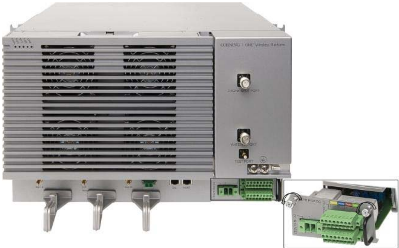
Figure 4-10. Extracting PSM from Chassis
